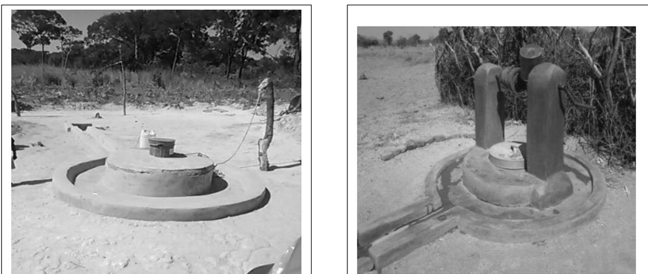
Photo 3 and 4. Improved Self-supply. Basic levels of improvement in Zambia and Zimbabwe respectively
