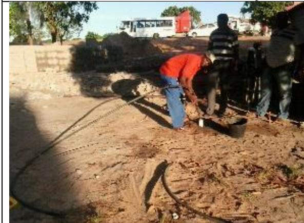
Making a Tube well with the Mzuzu drill. After a first hole with the Soil punch the casing is placed and lowered by using a Tube bailer which pumps out sand inside the casing.
