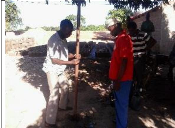
Making a Tube well with the Mzuzu drill Method, The first 3 to 7 meters is made with a Soil punch
