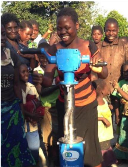
Figure 7. The first LifePump in Malawi was installed November 2013. The borehole was too deep for an Aridev and was declared dry until the LifePump arrived and could reach the water.
